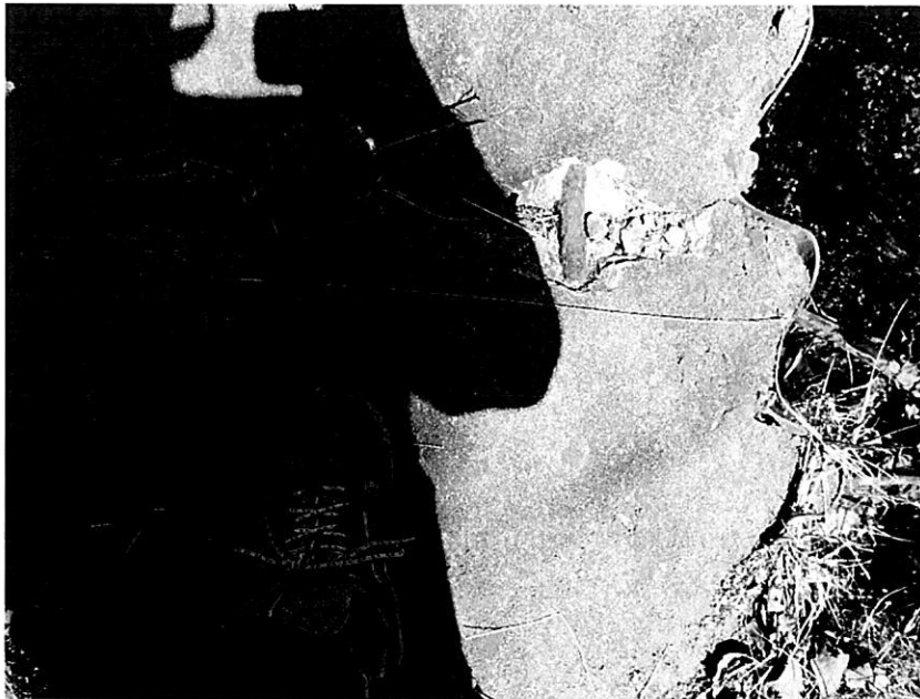
Photo 13 – Head Wall Exposed rebar
