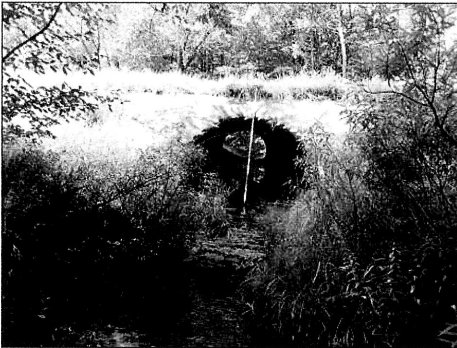
Photo 4 – Right Elevation (Downstream)
