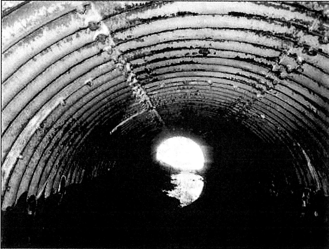
Photo 7 – General View of Underside. Looking Left
